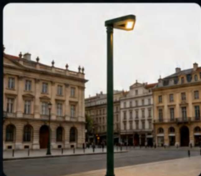
Urban Road Lighting
